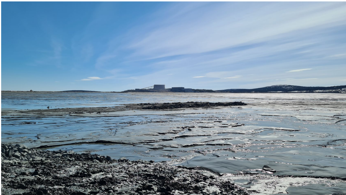
Figure 1: Tailings storage facility (TSF) at Aitik mine site, northern Sweden. The image shows mine waste in the form of slurrified tailings material that has been pumped into the open air tailings storage facility, after the mineral ore is processed. Aitik is one of the Boliden-owned mines that will form part of the PhD project, to establish a methodology for establishing and monitoring carbon capture and sequestration (CCS) through in-situ mineral carbonation in the TSF.
