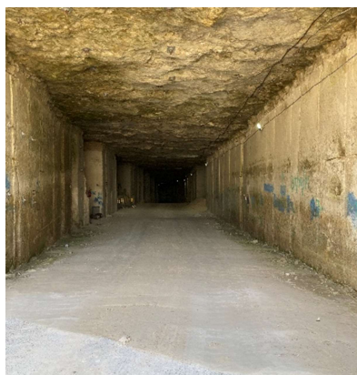
a. Cessation of Albion Stone mining activity in underground space
